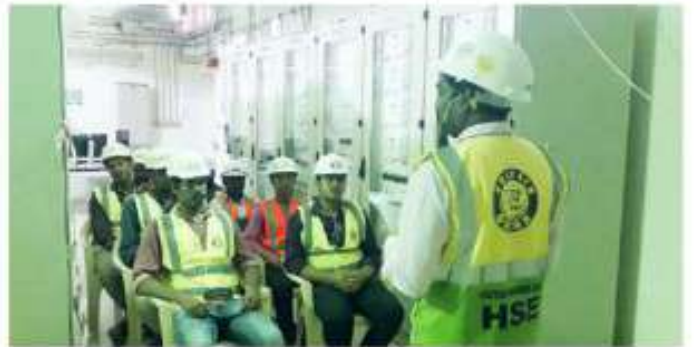
Doha Super Substation
