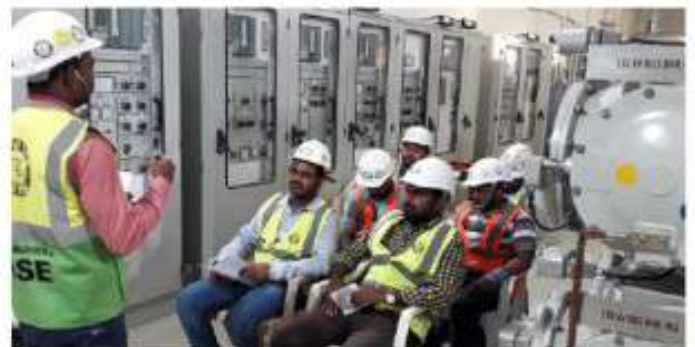
Jeriyan Jenaihat-1 Substation
