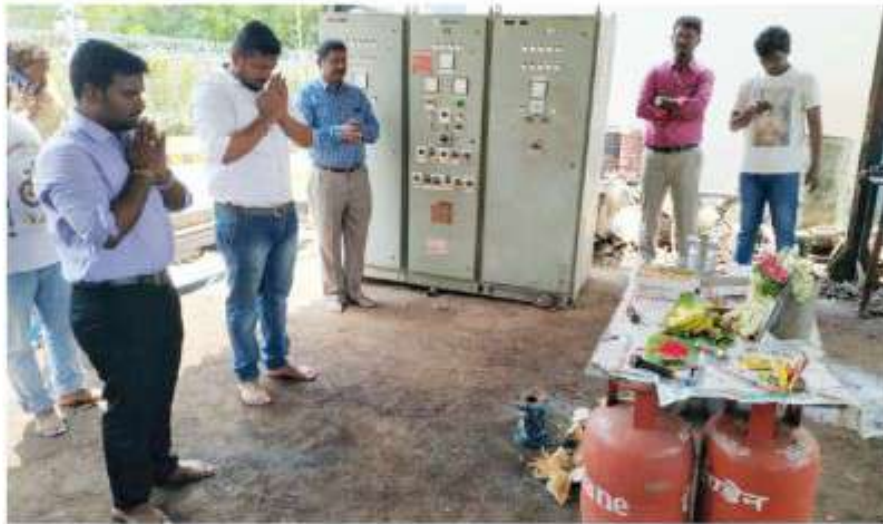
IOCL, Indane Bottling Plant, Ida Phase 3, Cherlapally – Commencement of Yokogawa Project Site.
