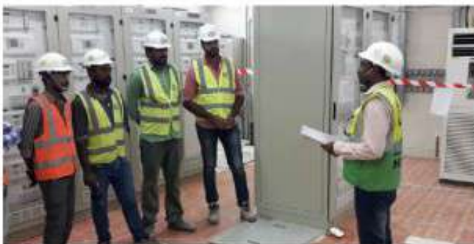
Lusail West-2 Substation
